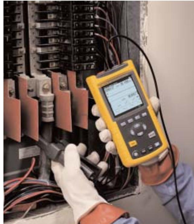
If intermittent voltage sags are suspected, start at the panel to isolate the cause of sags: Are the sags the result of loads on the same branch circuit or are they caused by loads elsewhere in the distribution system (including utility-generated sags)? We can start to isolate the source of the sag with the use of a handheld dual channel instrument with recording capabilities, such as the Fluke 43B Power Quality Analyzer. This helpful tool can trend both voltage and current simultaneously.
