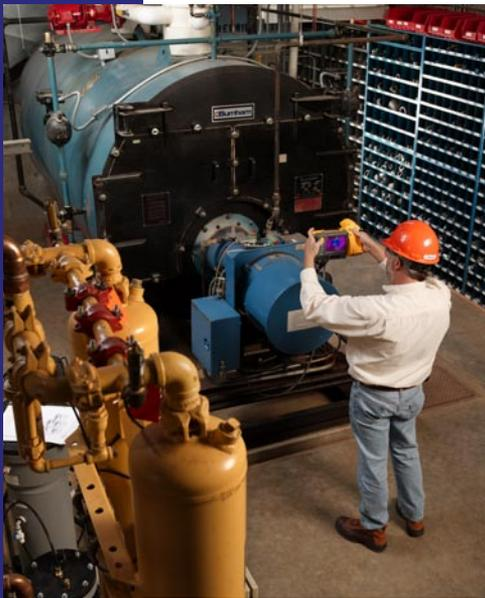
The purpose of a PdM program is to detect and prevent imminent failures before they occur to avoid the shutdown of critical equipment. One especially powerful tool for monitoring the condition of furnaces and boilers is thermal imaging, which captures two-dimensional images of the temperature profiles of objects. Thermal images can reveal potential points of failure in furnaces and boilers and help extend the life of their refractory insulation.
